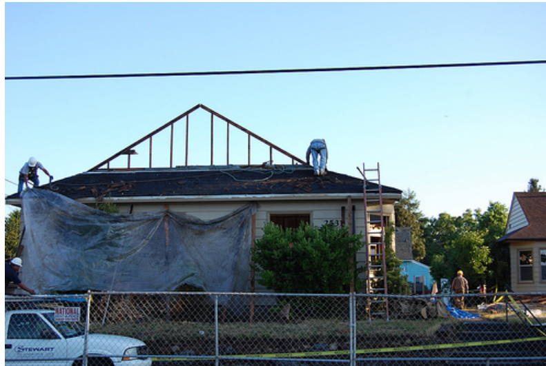
Figure 11. A deconstruction job in progress.
