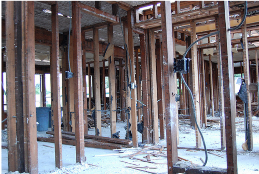
Figure 14. Building under deconstruction, down to the studs.
