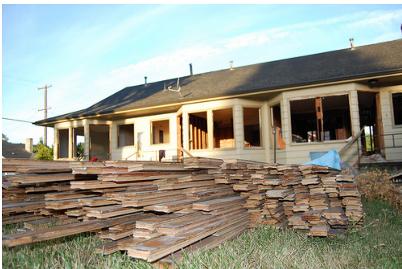
Figure 13. Salvaged flooring, sorted on the lawn of a house undergoing deconstruction.
