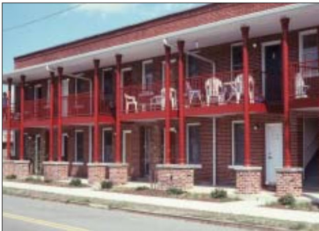
This 1904 building was renovated into one-bedroom rental apartments.
