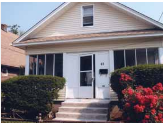
CDC of Long Island's first fully completed house under the WRAP (weatherization, rehab, and asset preservation) program, part of its insurance partnership under the loss-prevention component.
