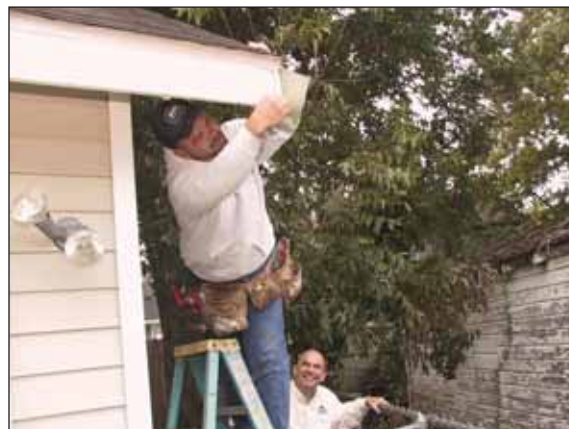
A Sears technician replaces siding on a resident's home.
