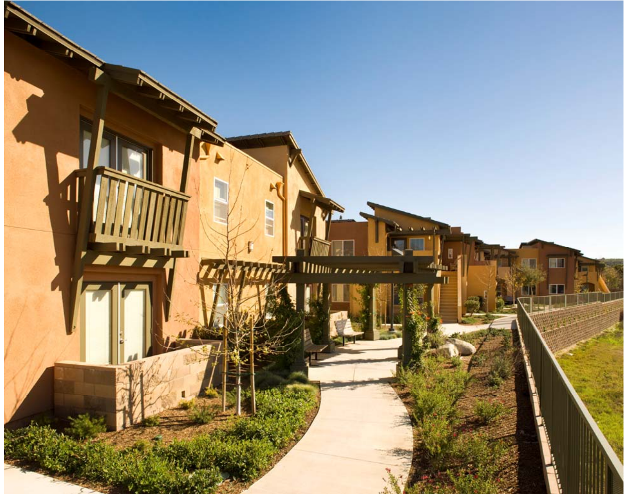
425' retaining wall along FEMA floodway
