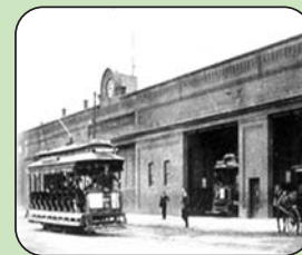
Turning a trolley barn into affordable housing.
