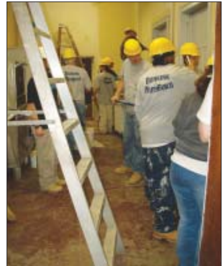
A western New York group at its job site.
