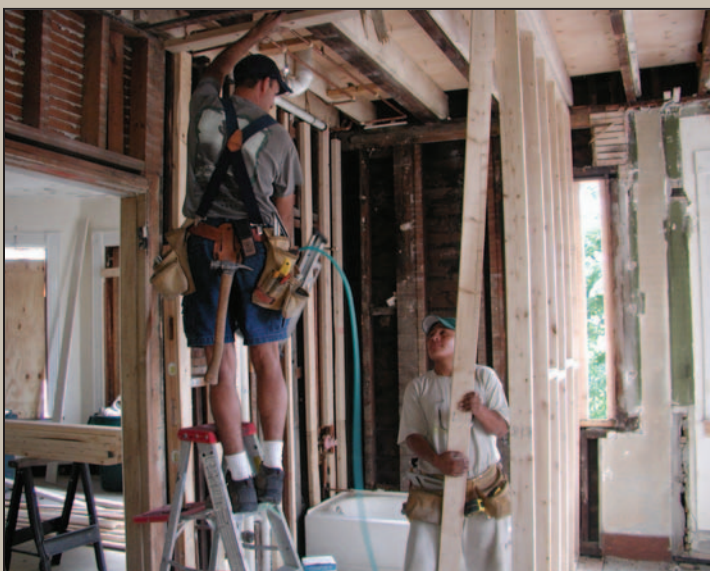
A Jackson Terrace bathroom in the making. COURTESY LAWRENCE COMMUNITYWORKS
