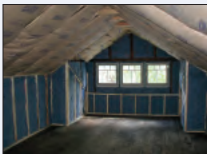
Adding extra insulation.
