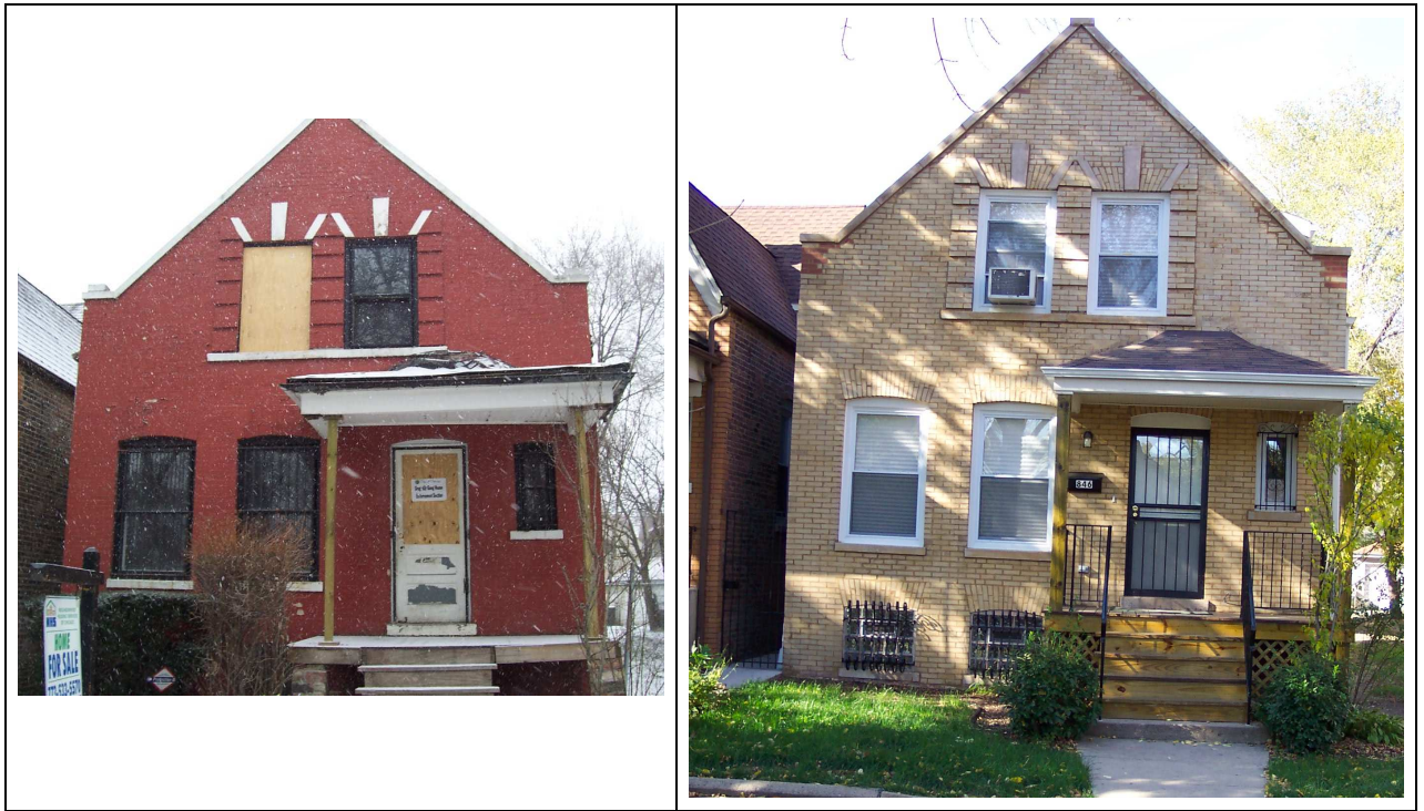
Figure 4. A Successful Rehab Through the Troubled Buildings Initiative II
